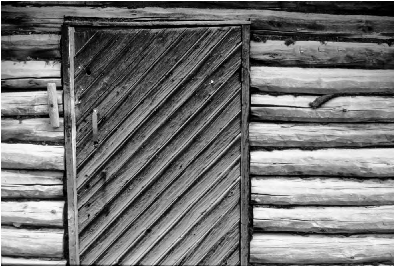
Cabin door at Ft. Egbert, Eagle, Alaska, 1983. © R. Drozda.
