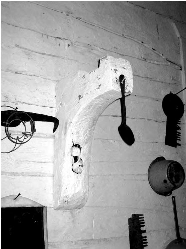
Figure 10: Roof bracing made of driftwood stump, Napaimute
