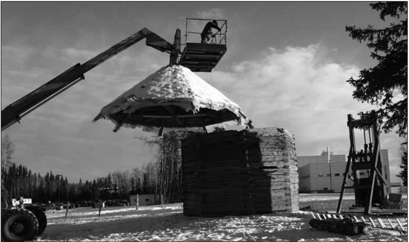
Figure 4: The spruce pole roof from 1982 being removed from the blockhouse in 2010.
