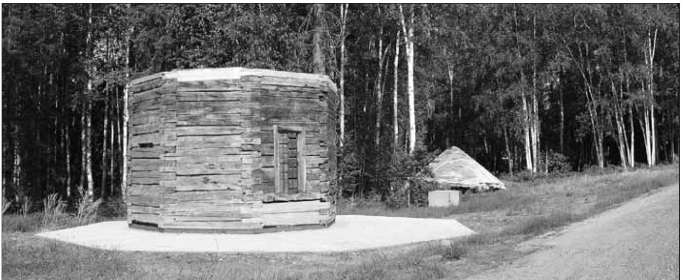
Figure 5: The blockhouse and roof (in background) on the new foundation.
