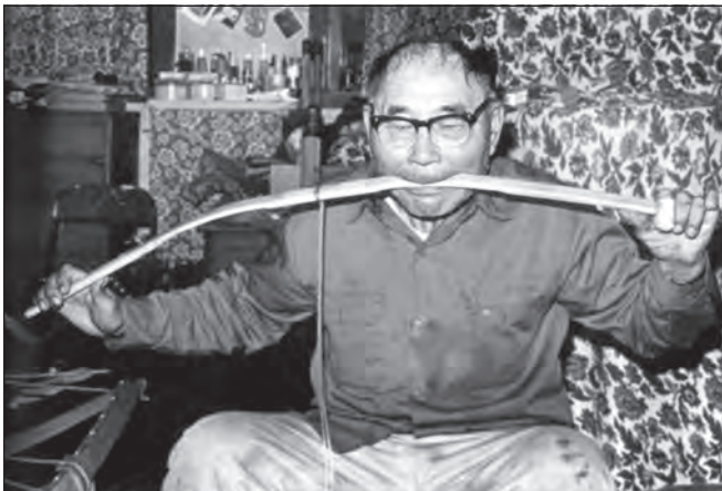
Fig. 4: Dick Bunyan, Rosalie's father, bending a kayak rib, 1976. Photograph by David Zimmerly.
